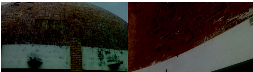
Figure 5. Conservation state of Dome 1 with coloration or discoloration, missing part, moist areas, scaling and efflorescence.
